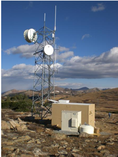
ReliOn fuel cell powering cell site
